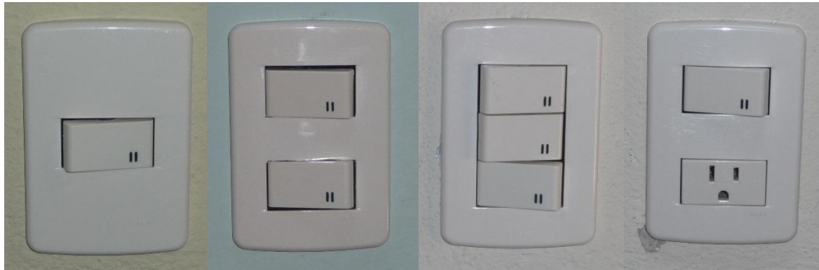
Figure 2-13 New Style (Modular) Switches and Outlets
