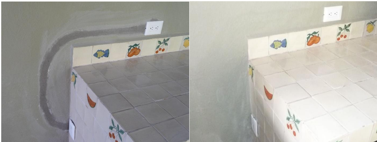
Figure 4-20 Installing New Circuit Step 4
