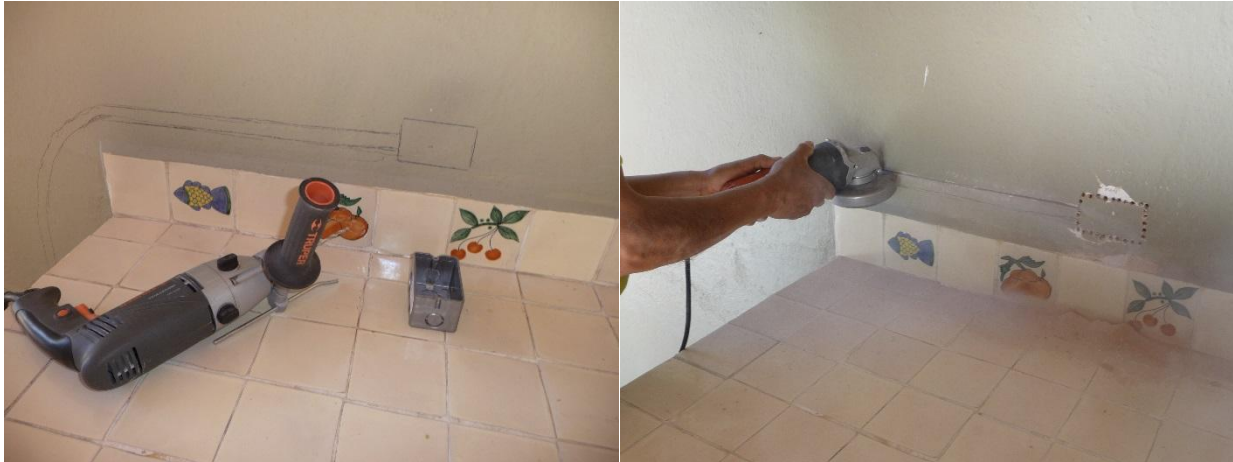
Figure 4-17 Installing New Circuit Step 1
