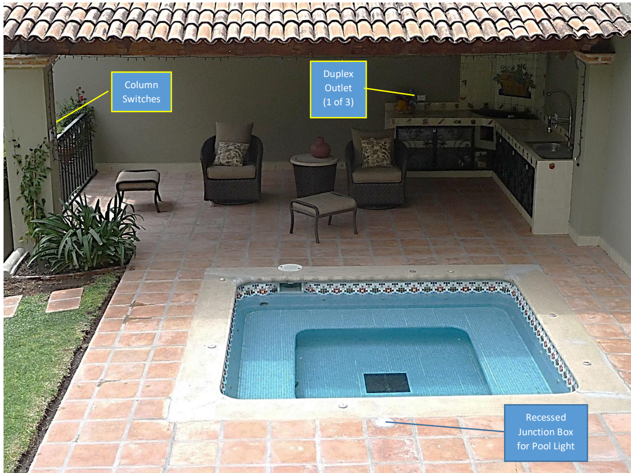
Figure 9-17 Rewired Upper Pool Area
