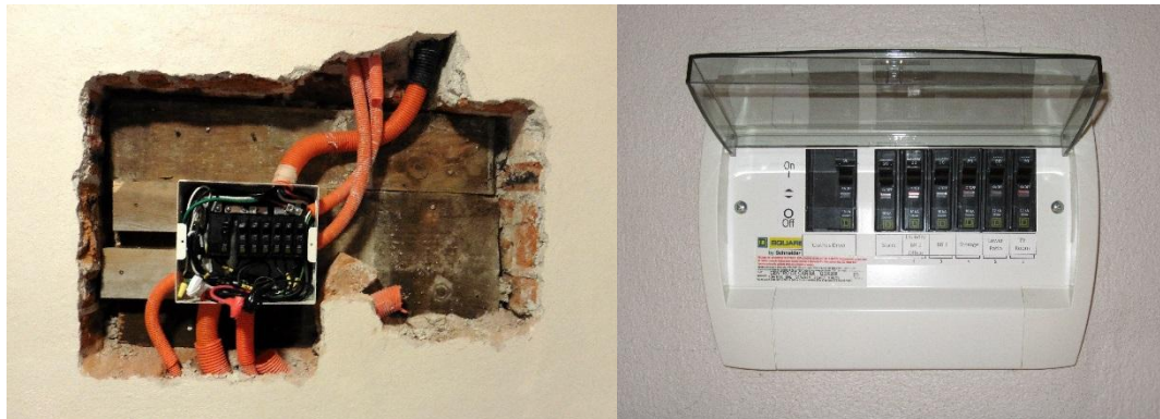
Figure 12-12 QOX206 Subpanel which Replaced Store Room Subpanel and Knife Switch
