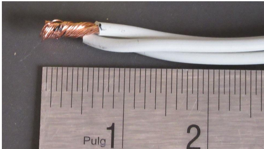
Figure 2-11 Wires Re-cut for Wirenut
