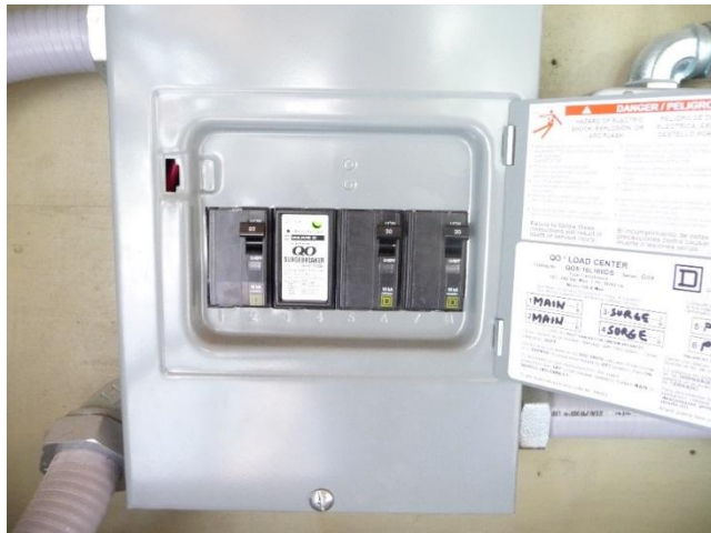
Figure 4-8 Surge Protector Installed in Entry Panel
