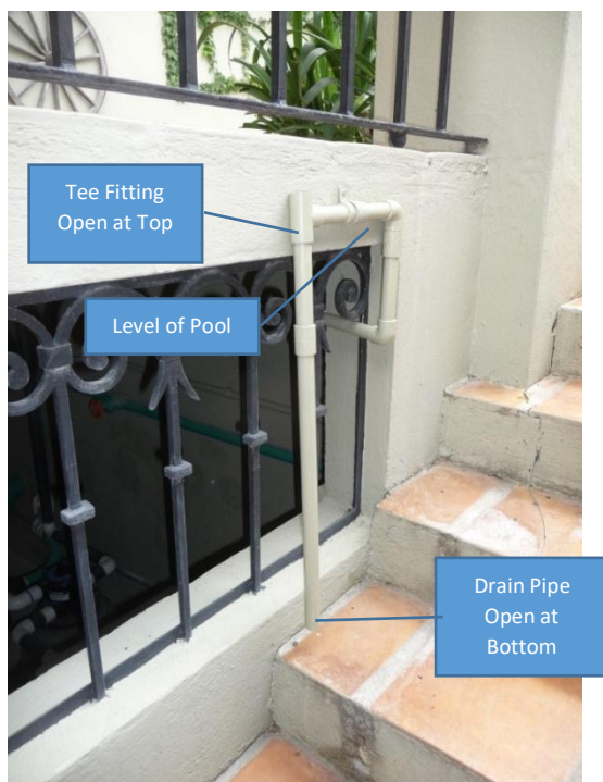
Figure 9-19 Drain Pipe
