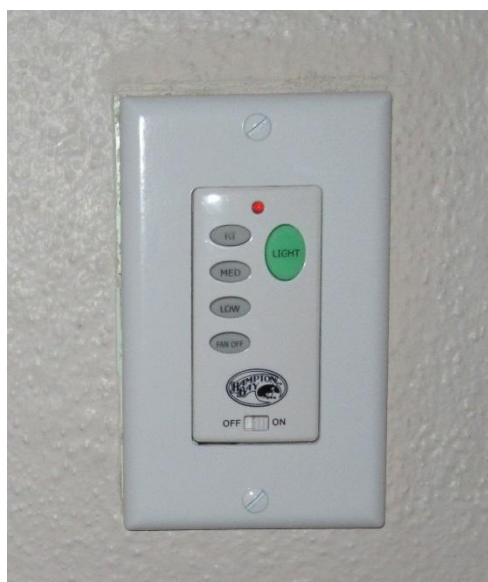
Figure 12-21 Wall Mounted Fan Control Used in Colibrí
