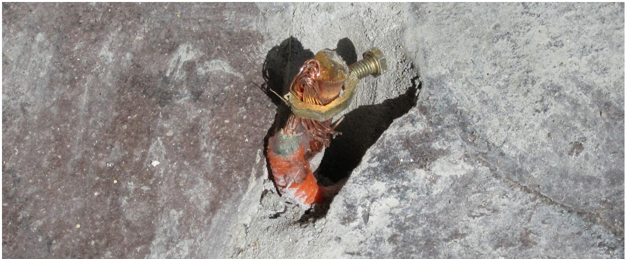
Figure 10-16 Earth Ground for Meters
