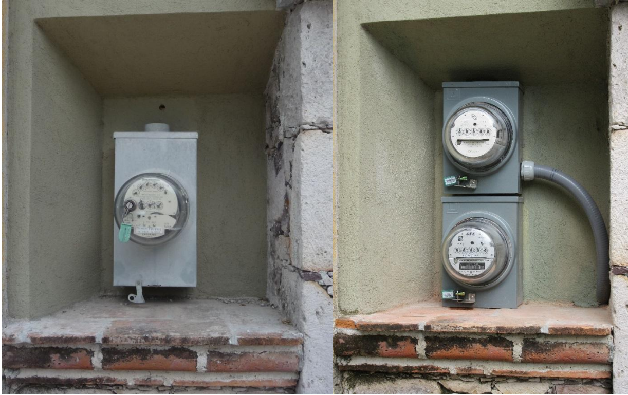
Figure 10-15 Original Erres Meter (Left) and New Meters (Right)
