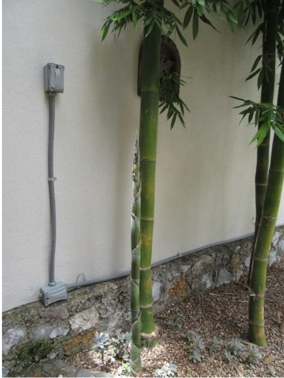
Figure 12-7 Waterproof Conduit and Boxes for Timer and Outlets at Colibrí
