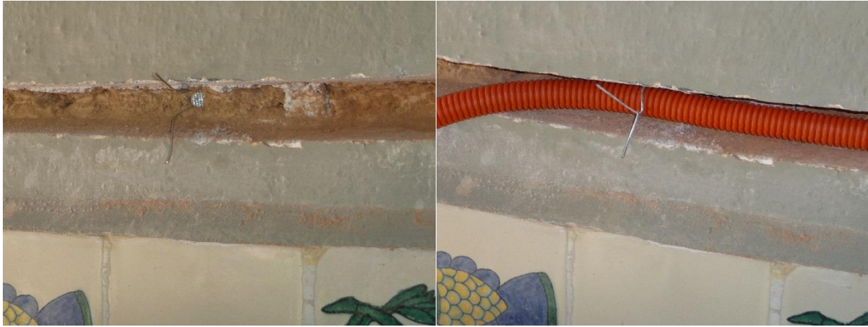
Figure 4-19 Installing New Circuit Step 3
