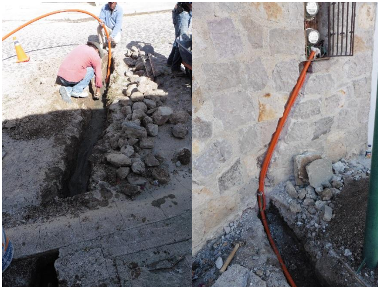
Figure 12-15 Installing New Conduit between Meters and CFE Junction Box
