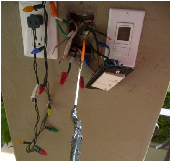
Figure 9-16 Pulling New Green Wire through Conduit P at Column Switches
