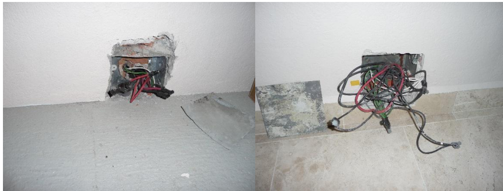
Figure 12-9 Hidden Junction Boxes in Garage (Left) and TV Room (Right)
