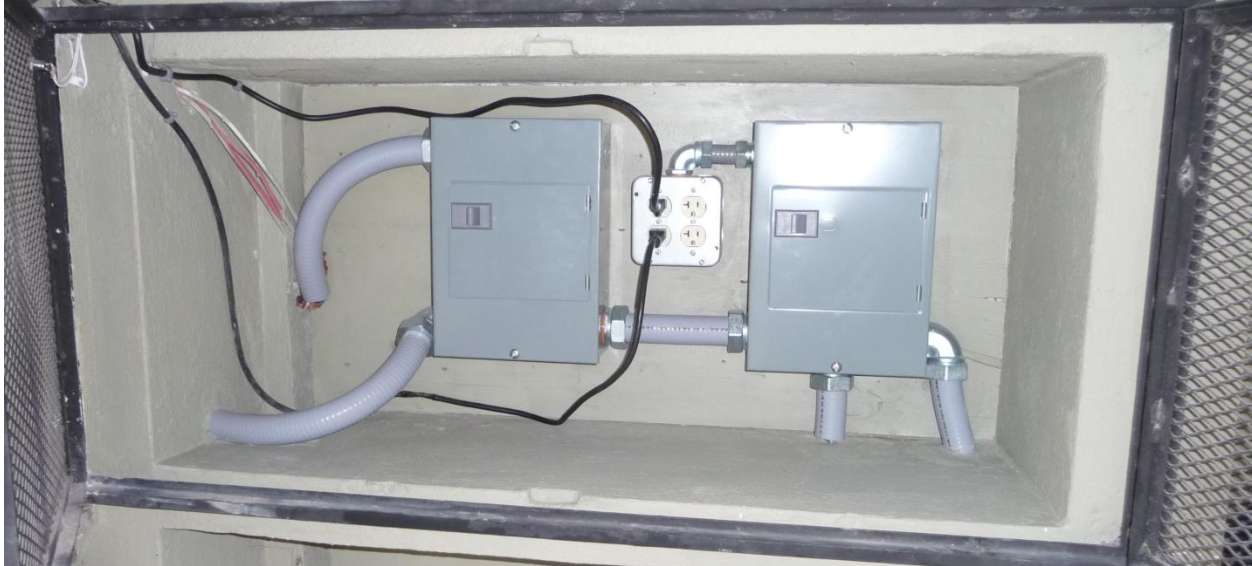
Figure 10-9 New Entry Panels with Covers
