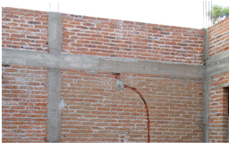
Figure 2-7 Wall with Castillos and Cadenas. Note Electrical Box and Conduit
