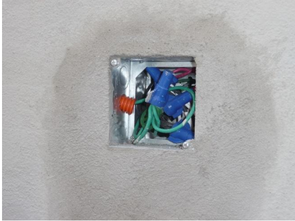
Figure 12-5 Kitchen Junction Box after Rotating and Extending to Outer Wall
