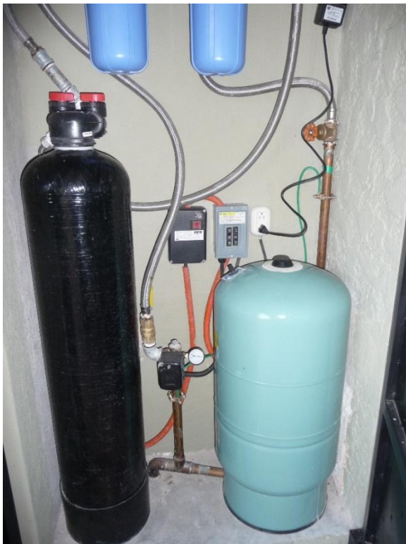
Figure 4-6 Ground Wire at Filter Pump
