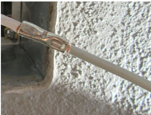
Figure 12-6 Butt Splice Used to Extend Conductors on Kitchen Junction Box
