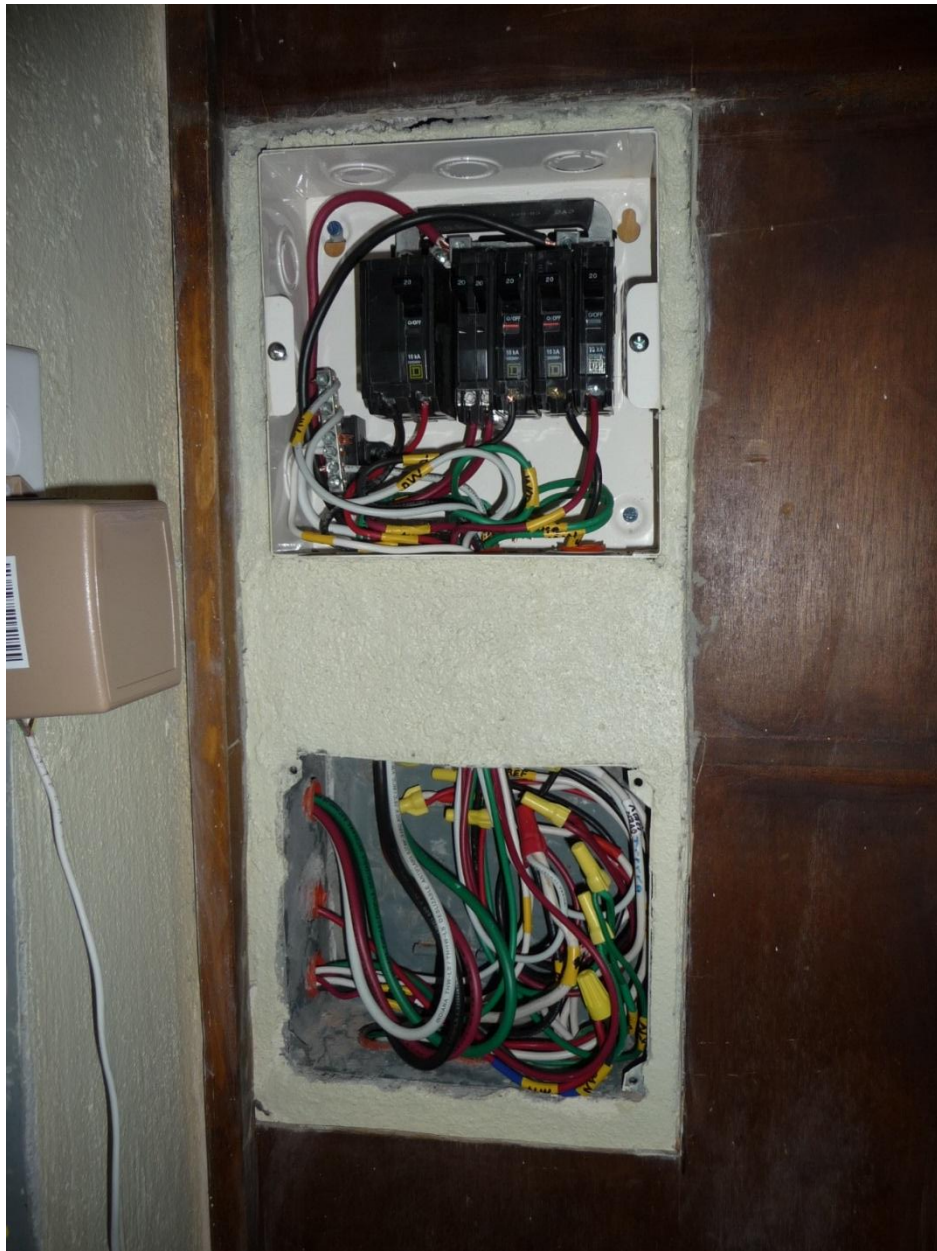
Figure 10-13 New Appliance Subpanel after Wiring
