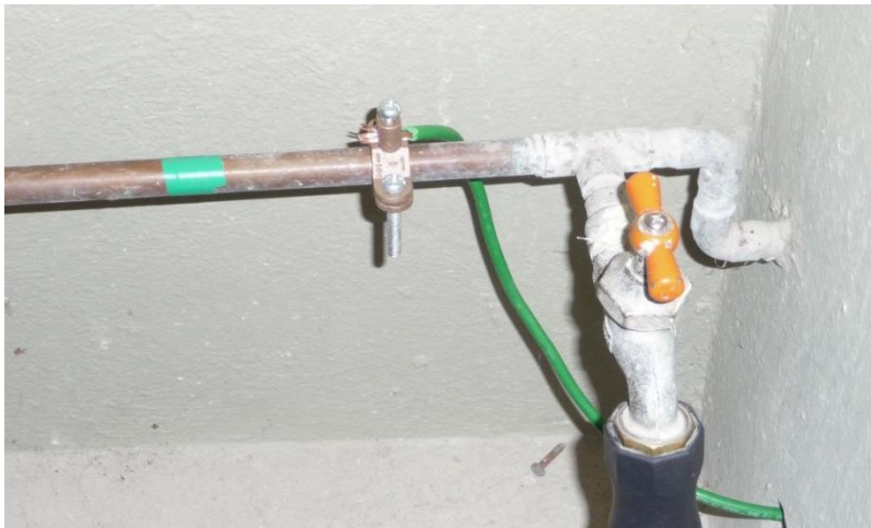
Figure 4-4 Ground Wire between Entry Panel and Main Water Pipe
