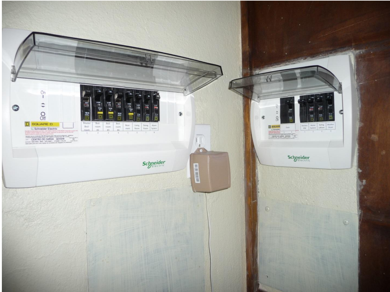
Figure 10-14 New House and Appliance Subpanels with Junction Boxes Covered Below
