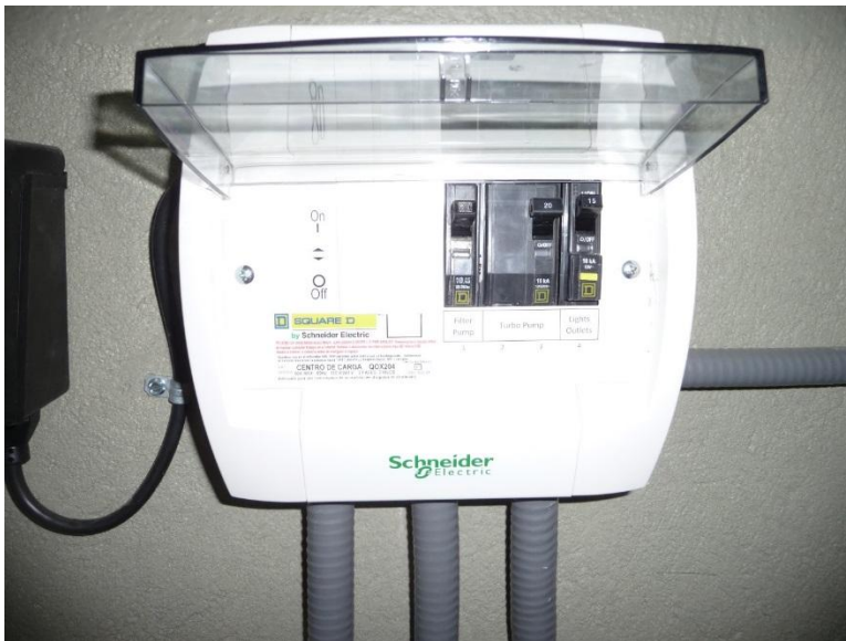
Figure 9-14 New Subpanel for Pool with Timer on Left
