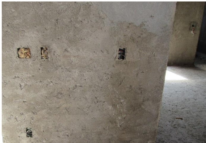
Figure 2-8 Wall after Rough Coat of Plaster
