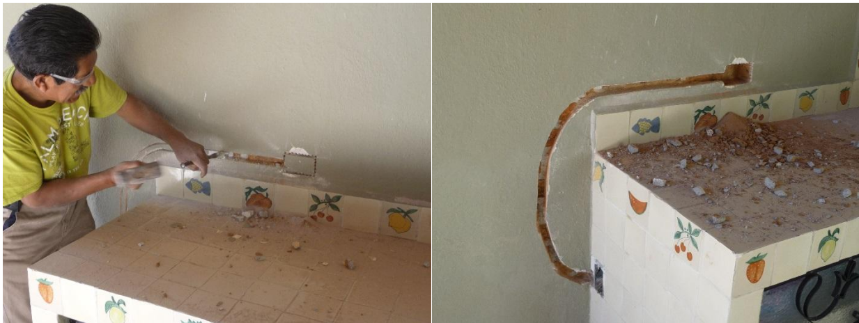
Figure 4-18 Installing New Circuit Step 2
