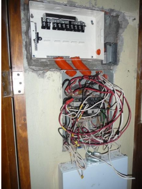
Figure 10-10 New House Subpanel Installed above Original House Subpanel
