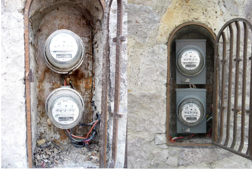
Figure 12-16 Before (Left) and After (Right) Meter Installation
