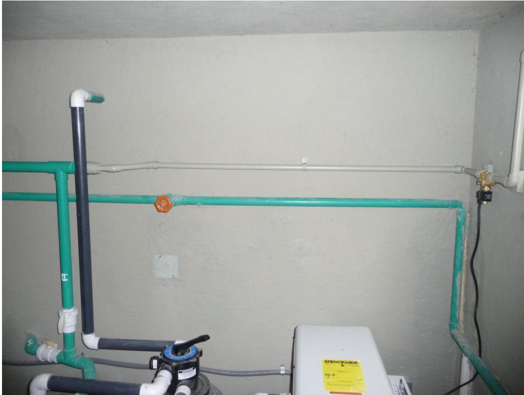
Figure 9-18 Overflow Pipe Connected to Pump Inlet
