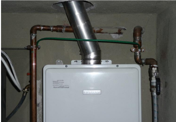
Figure 4-5 Ground Wire at Water Heater
