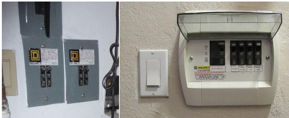
Figure 12-13 Original and New Garage Subpanels
