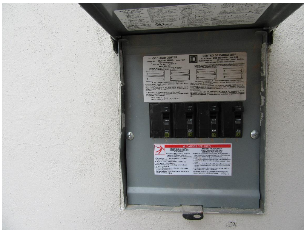
Figure 13-3 Soledad Main Breaker Panel – The 70 amp main breaker is on the left, the two 50 amp subpanel breakers are in the middle and the 20 amp water pump breaker is on the right.
