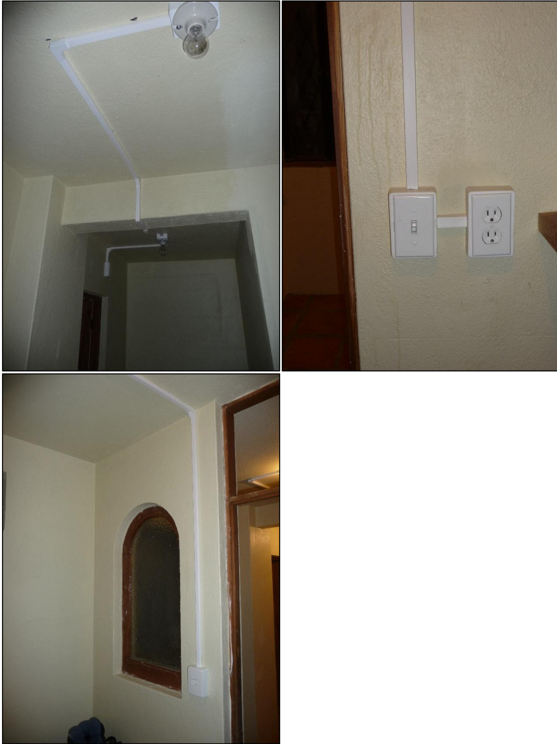
Figure 11-3 Wire mold raceway and boxes in basement
