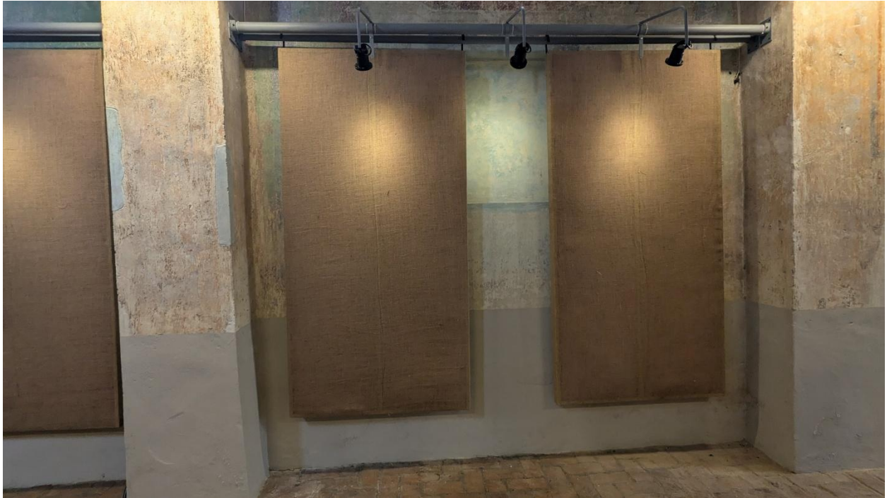
Figure 18 Panels Mounted on Rails
